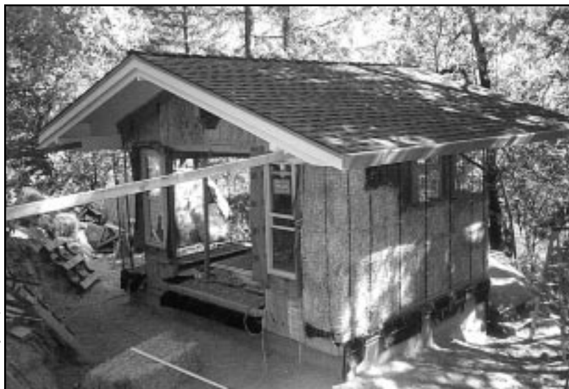
Straw-bale kuti under construction
